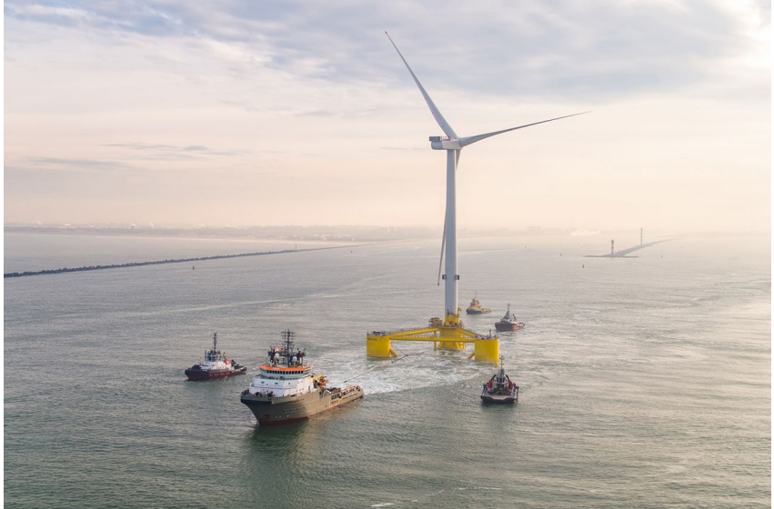
Boskalis AHV towing floating turbine to site: Source: Boskalis.
