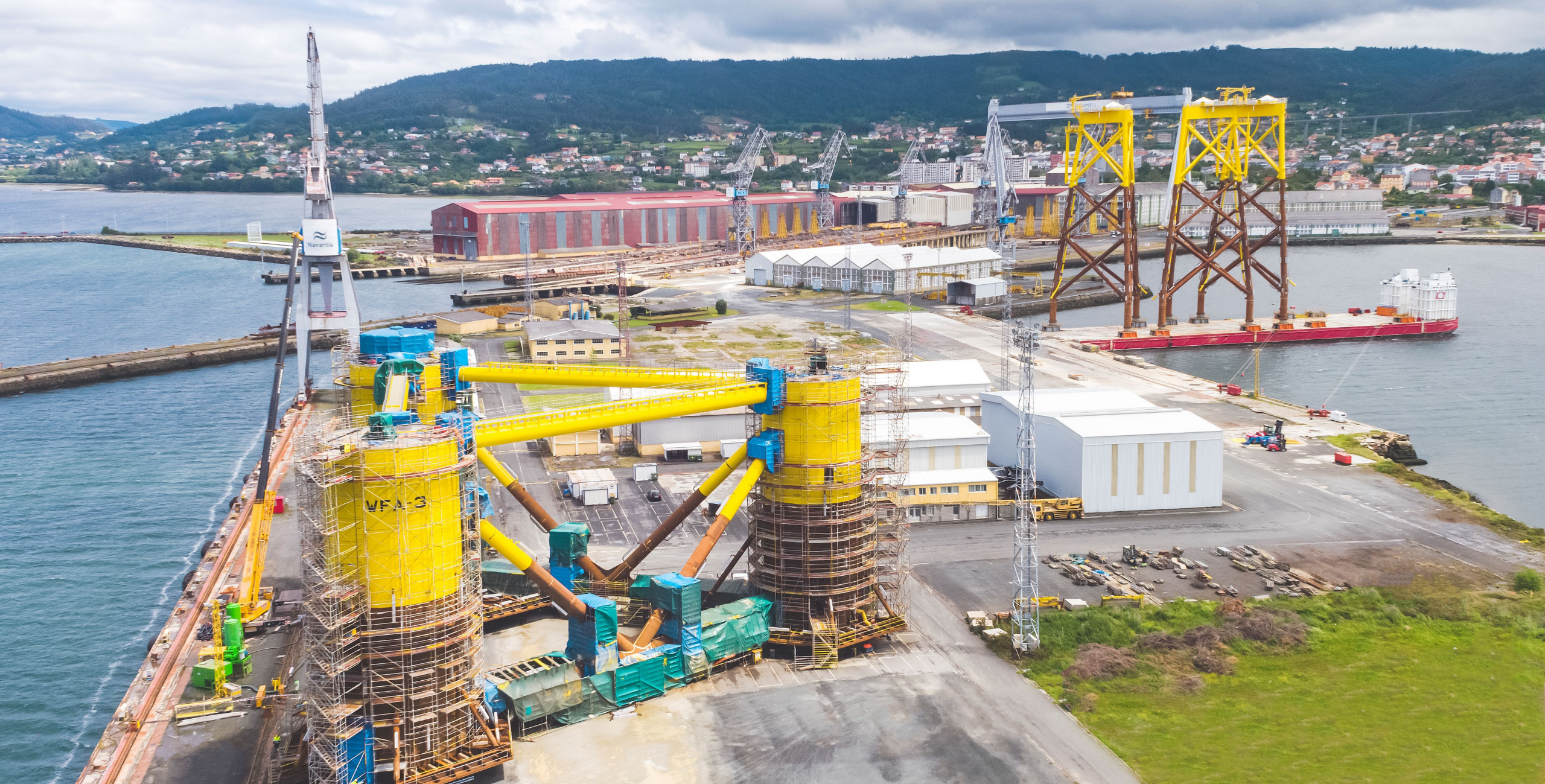
Source: Photo of the WindFloat Atlantic project courtesy of Principle Power/Ocean Winds (floaters designed for 8.3MW wind turbines – foundation of ~3.000 metric tons)
